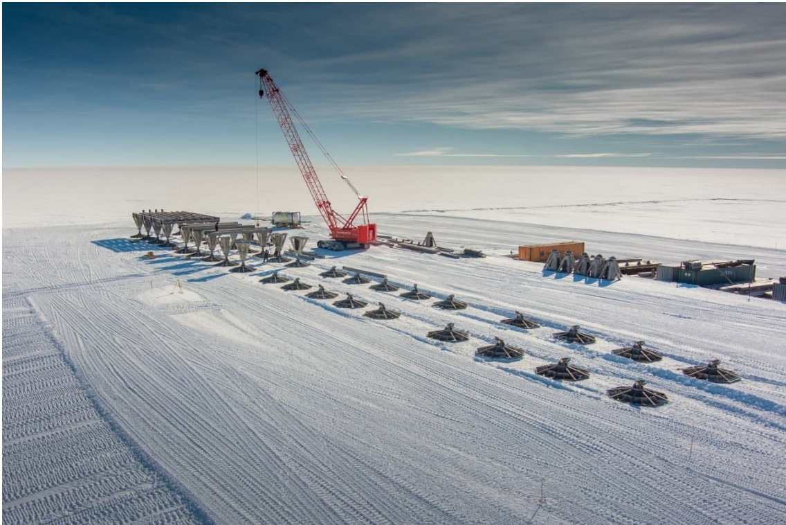
Figure 2 – Installation of ski-pillars and base platform
