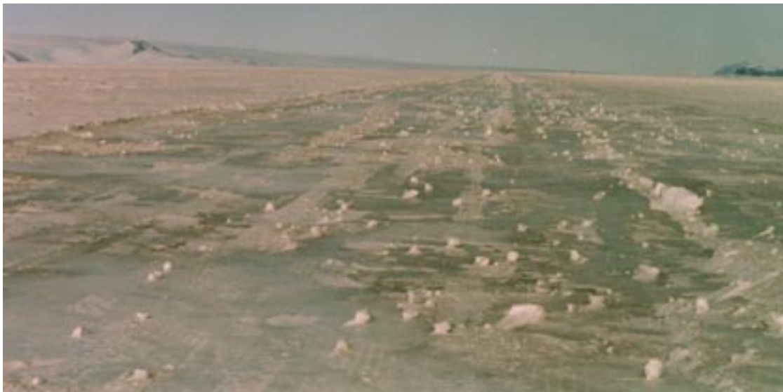
Figure 39. Ice surface following initial grading.
