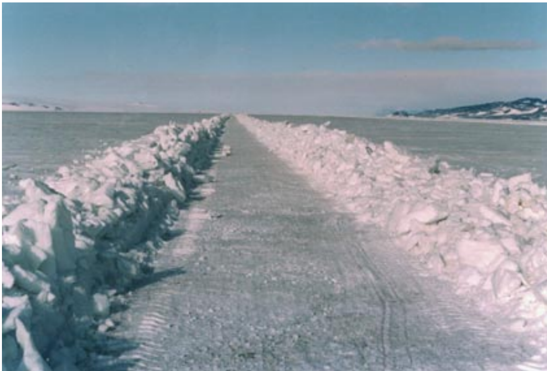
Figure 32. Ice surface following initial snow stripping.
