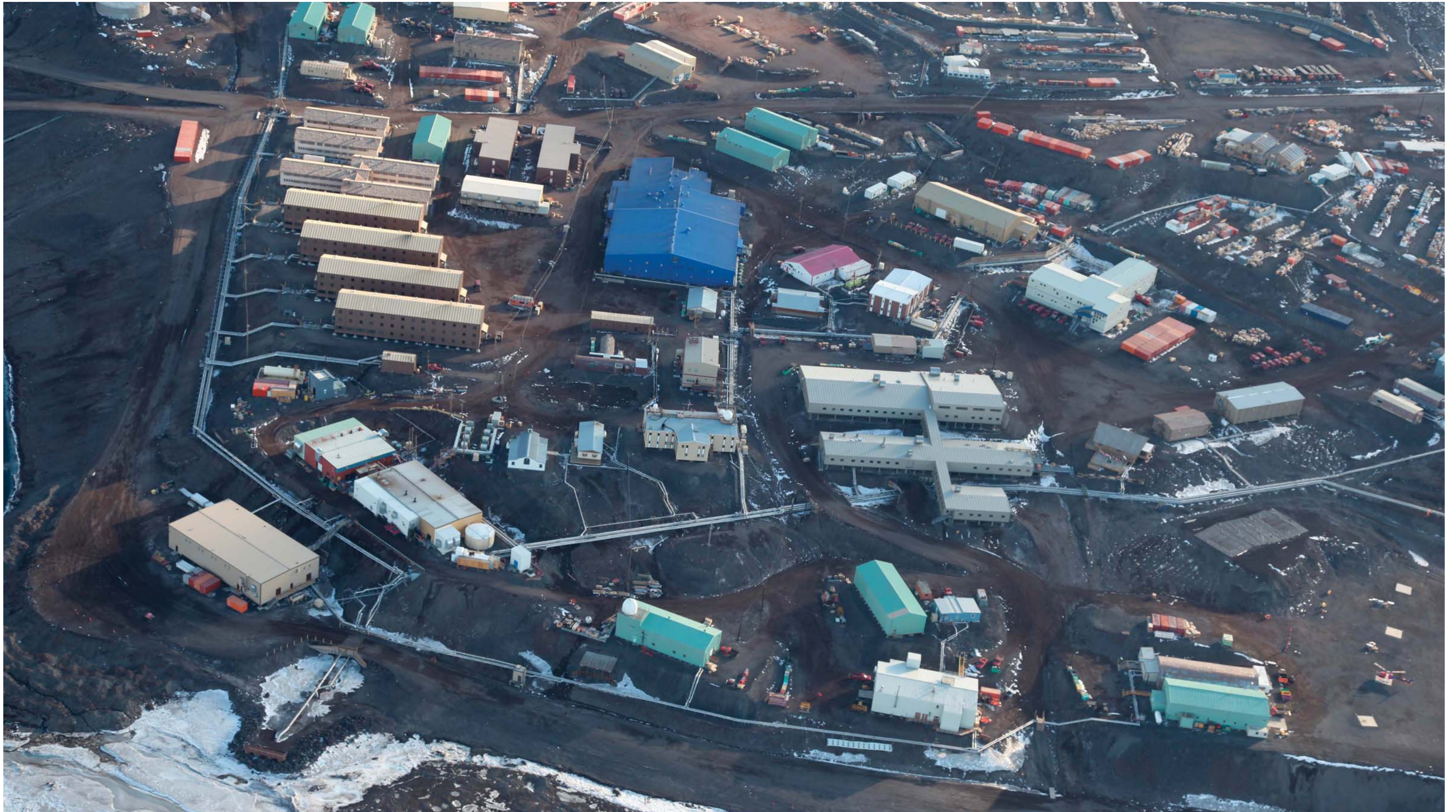
EXISTING MCMURDO STATION
