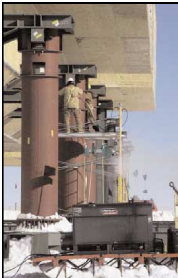
At left, the footings under the main section of the new station have been settling faster than the staircase tower. Below, workers jack up the station in increments to bring the sections level with each other.
